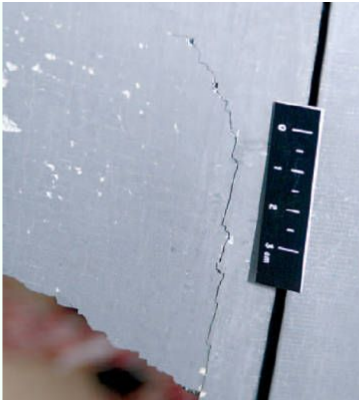
Numerous cracks were also noted in RCC Panel 8.
